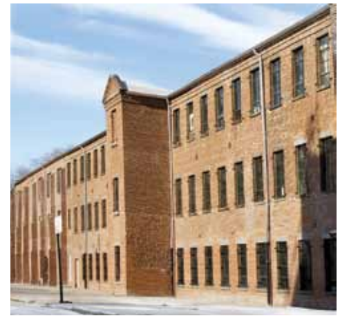
Figure 5: 221 McKibbin Street Industrial Center was recognized with an Historic Preservation Award in 2009.
