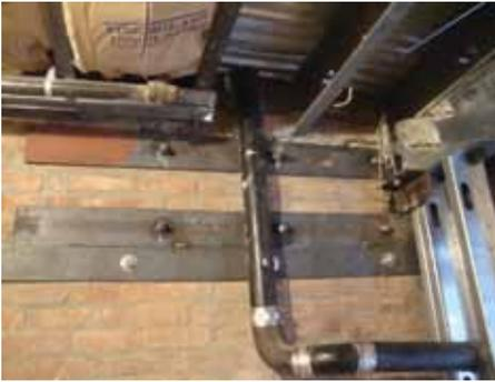
Figure 5: Steel strap ties on wall.
