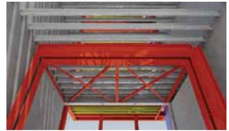
Figure 6: Offset of moment frames at second floor.
