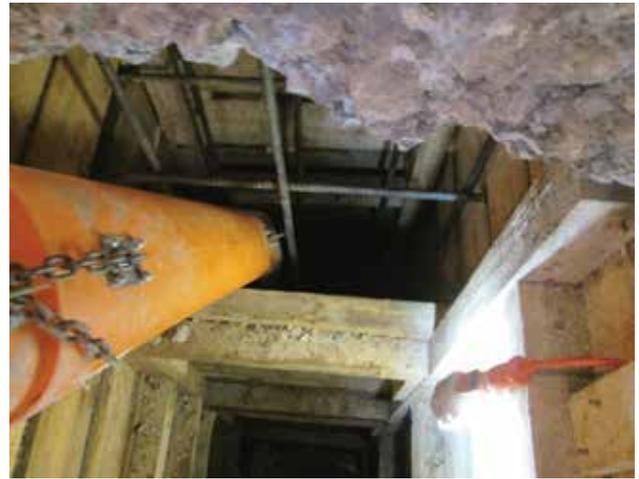
Figure 1. Installing an underpin beneath foundation.
